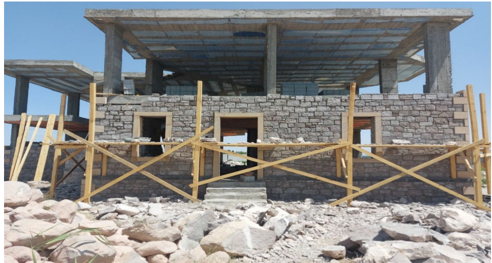
Fig. 2 House built using andesite stone in Iğdır province, Türkiye
